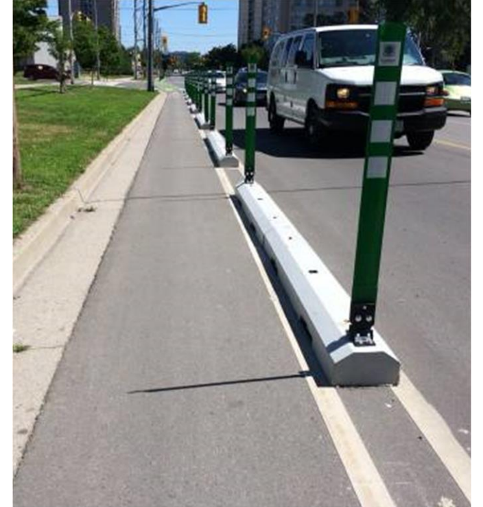
PRECAST CONCRETE CURBS WITH FLEXIBLE BOLLARDS
